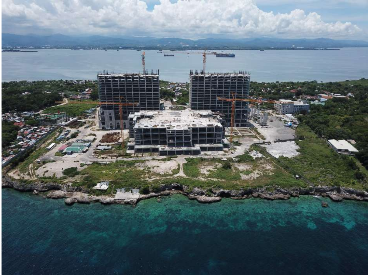
Emerald Bay under construction as of 9 September 2020
